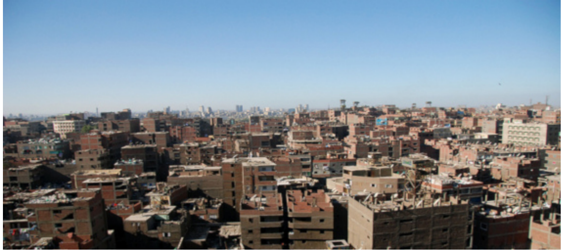
Unfinished buildings in Cairo (photo by Kim Eun Yeul via World Bank Photo Collection .(Flickr
